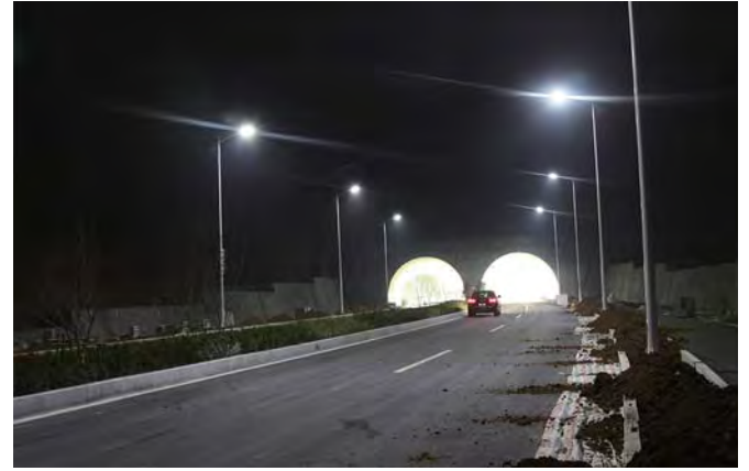
- for Road, China
